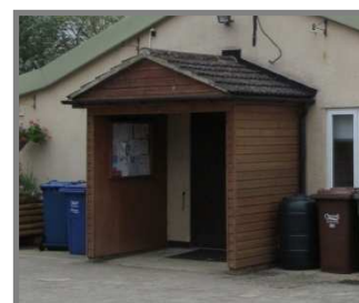
A door could be added to the front porch where users could open the front door, enter the porch, close the front door and then enter through the main hall door. This would help reduce draughts and maintain the indoor temperature.
