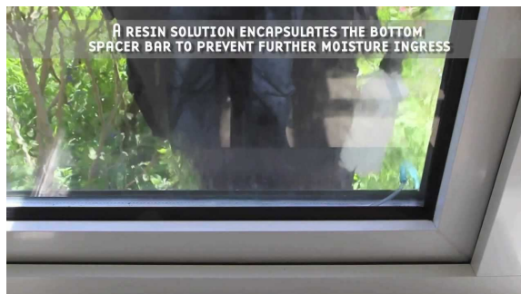
An example of how double glazed units can be repaired http://tinyurl.com/IWSolution
